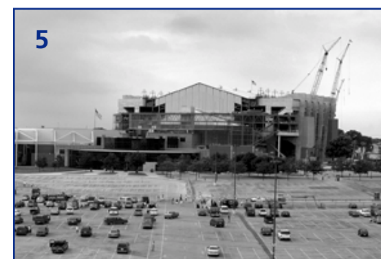
Raising the 1200-ton roof 41 feet, 10 inches on August 2, 2002, took just under five hours.
