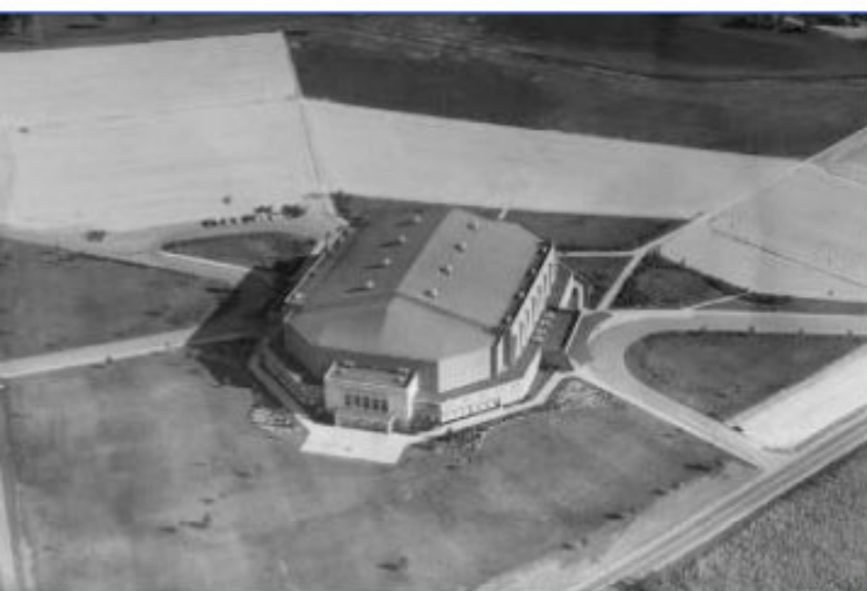
The newly constructed Memorial Coliseum in 1952 at the corner of Parnell Avenue and California Road
